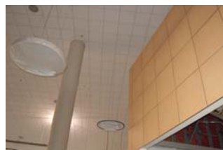
Ceiling and wall tiles installed in the Meeter/Greeter Hall.
