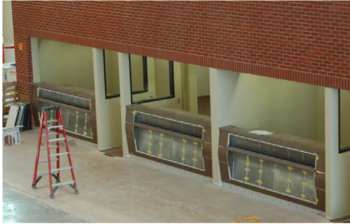
On right, the yellow tape is used during the assembly and installation of the counters' faces. At left, agencies will customize their shelving behind counter.
