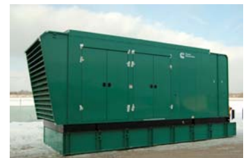
If power should fail, the terminal's new generator can support critical equipment, systems, and safety devices.
