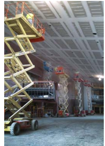
Tradesmen sand the arrivals lobby ceiling in the new terminal.
