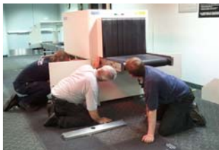
Technicians dismantle the x-ray machine for transportation to the new terminal.
